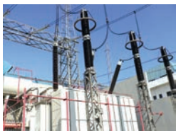
Power Generation (Contracted)
